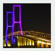
The main bridge using a cable stayed construction supported by the twin towers for about 140 meters. And the main bridge deck is using composite construction dor 2.4 meters thick.
